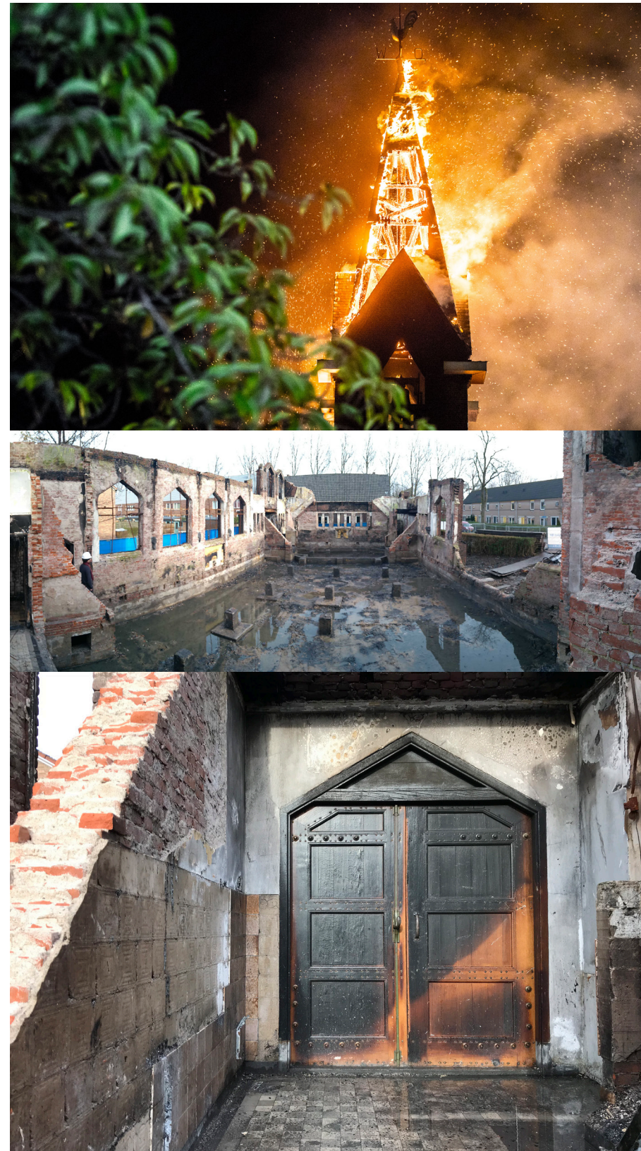
Fire on the 6th of August 2018 and aftermath | Julianakerk
