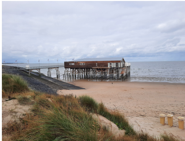
Figure 5.1: Strandclub Zee at the Brouwersdam beach, photo taken at approximately MWL (mean water level) (photo taken at 31-08-2020)
