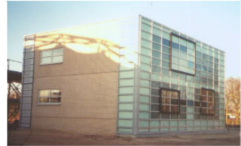
Figure 2.7: IFD trial module, Eindhoven University of Technology (Source: Gassel, 2003)
