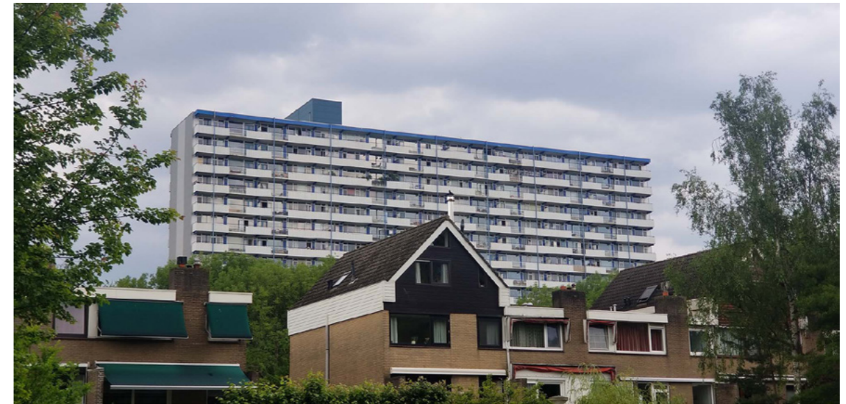
Figure 7.22 Menno ter braaklaan pedestrian view (Source: Author)
