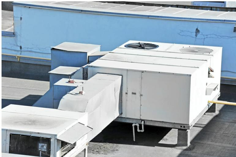
Figure 3.2: HVAC rooftop unit.<sup>4</sup>
