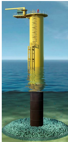
Figure 2.2: Monopile with transition piece and scour protection [61]
