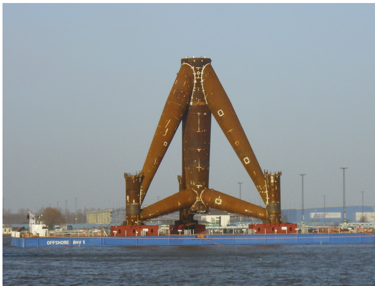
Figure 2.6: Tripod substructure to support offshore wind turbine
