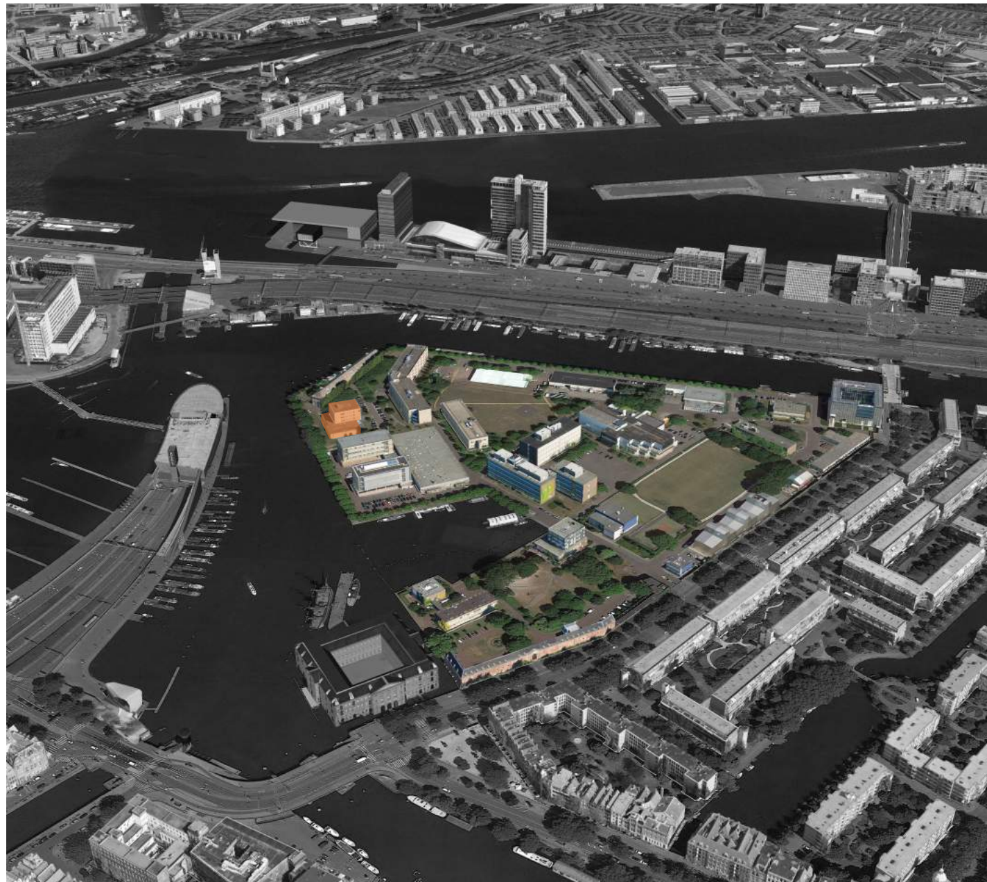
From shipyard and dock towards reclamation of the dock and construction of the IJtunnel
