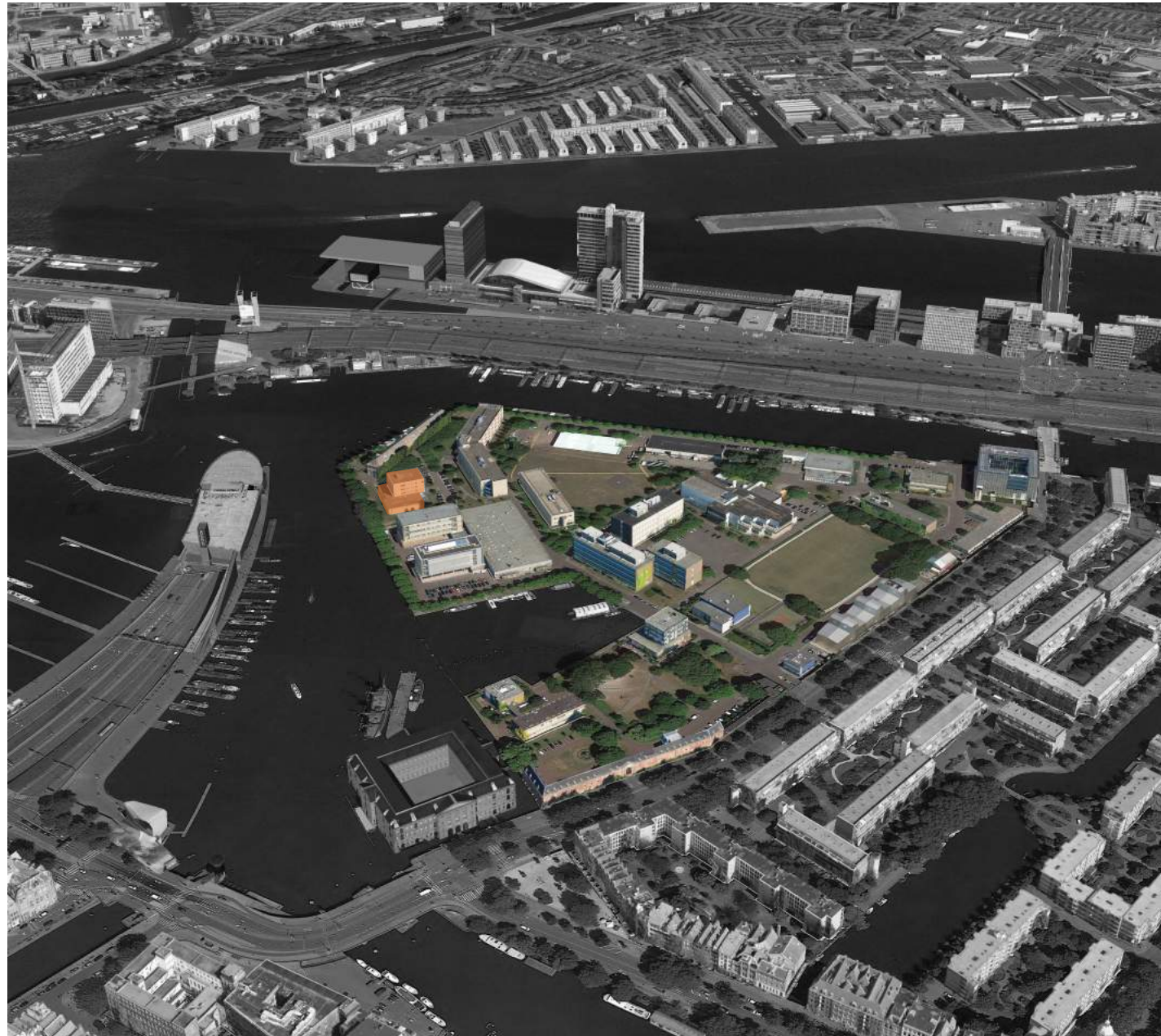
From shipyard and dock towards reclamation of the dock and construction of the IJtunnel
