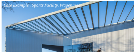
Case Example : Sports Facility, Wageningen For the new Sports Facility in Wageningen reusing materials in the new building was one of the focus points. A number of materials have been reused throughout the building, such as steel beams, wooden slabs, insulation, etc.
