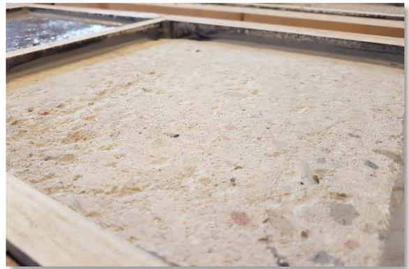
Figure 82: concrete surface treated by sanding
