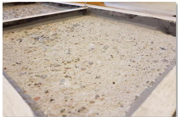
Figure 84: concrete surface treated by grit blasting
