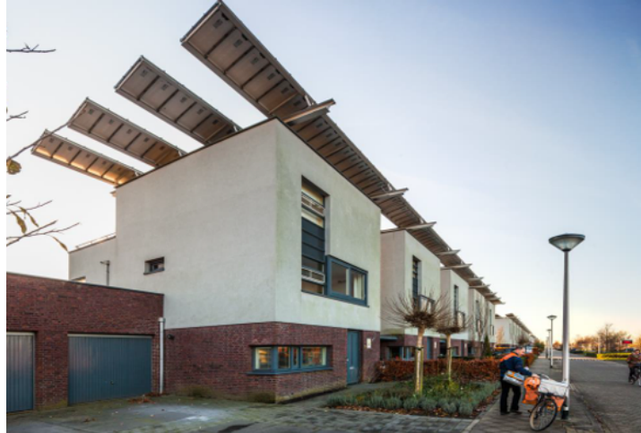
Figure 3.5: The NZEB in Rijsdijk, Etten-Leur [94].
