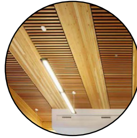
Rhythm of flat beams provides space for services
