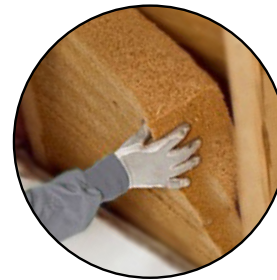
Wood wool insulation - eco friendly and sound-resistant
