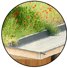
Expression of drainage system at roof's edge
