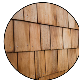
Solid balcony elements expressed with cedar shingles
