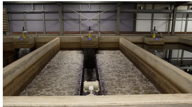
Figure 26: Unclogging of the sand filter (Waternet, 2018c)
