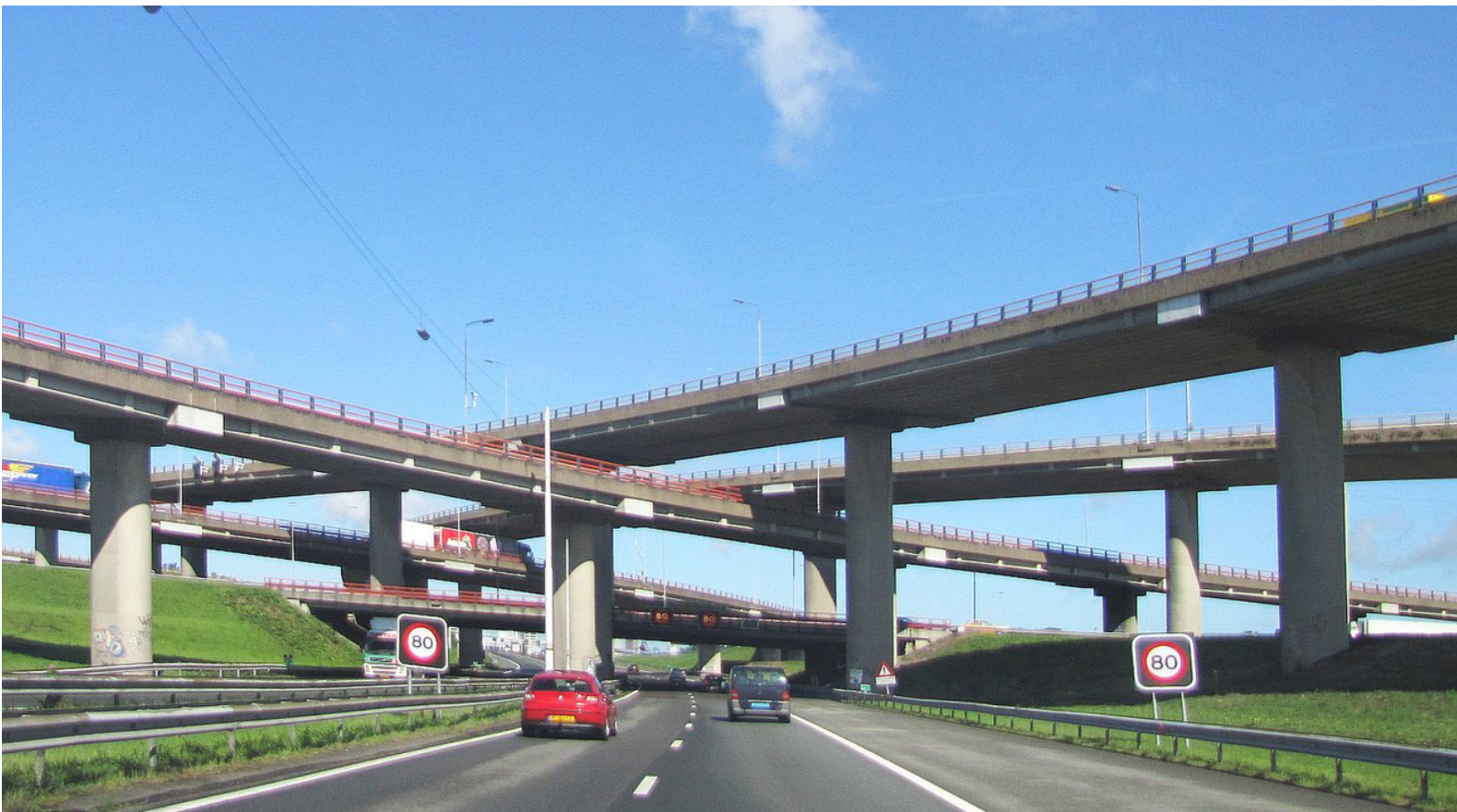
Part of the concrete bridges that have been identified by Rijkswaterstaat to be recalculated are the viaducts of the Prins Clausplein near The Hague in the Netherlands. Photo: Wolfgang Pehlemann
