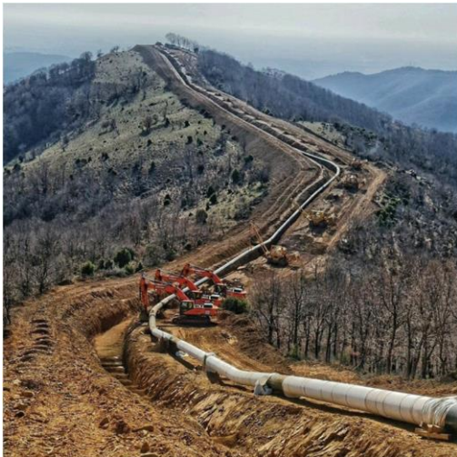
Figure 2.8a: Onshore Pipeline Lowered into a Trench [16]
