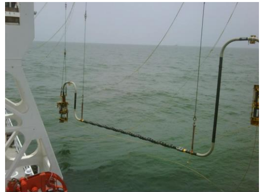
Figure 4.12: Jumper Installation [14]
