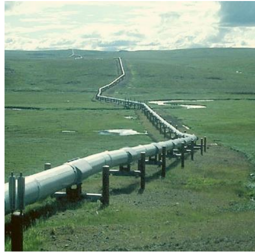
Figure 2.8b: Onshore Pipeline Installed Aboveground [22]
