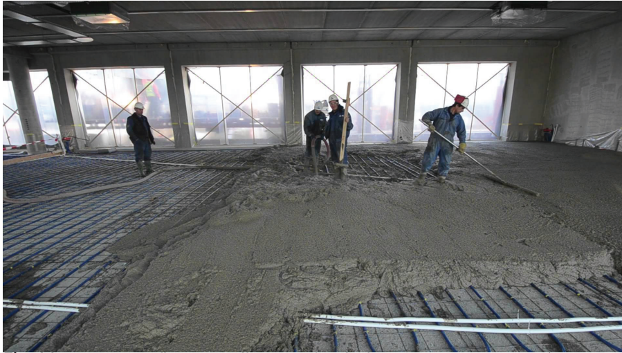
Fig. 38: Concreting flooring Lidl main office (FaberBetonpompen, 2012)
