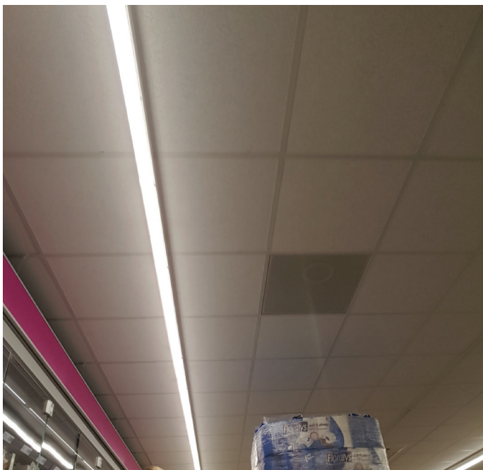
Fig. 102 Fig. 53: Drop ceiling, Lidl multatuliweg Delft (source: own image)
