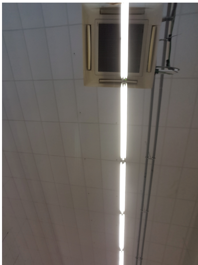
Fig. 60: Drop ceiling, Mercuriusweg Delft (source: own image)
