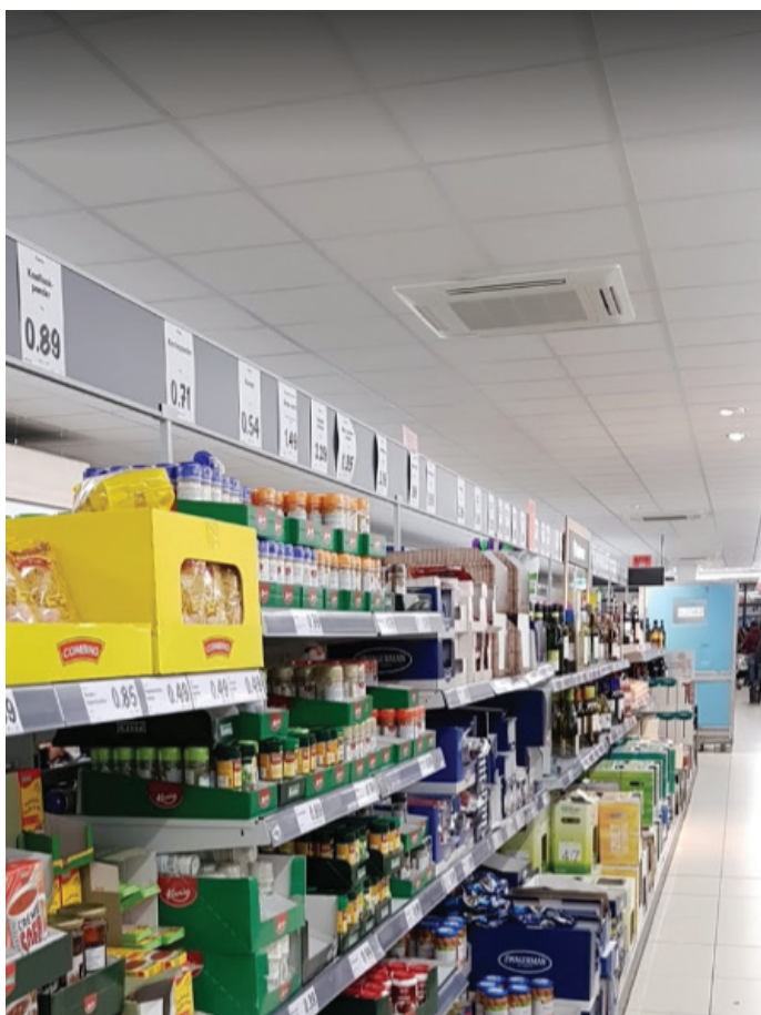
Fig. 59: Drop ceiling, Lidl Wesselsstraat Den Haag (source: own image)
