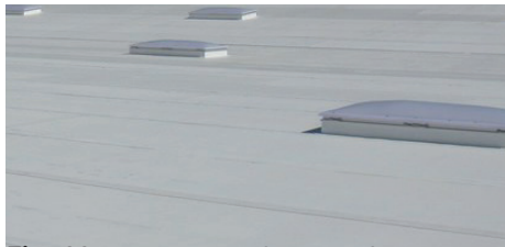
Fig. 68 : FPO roofing , element E (Mapeplan, n.d.)
