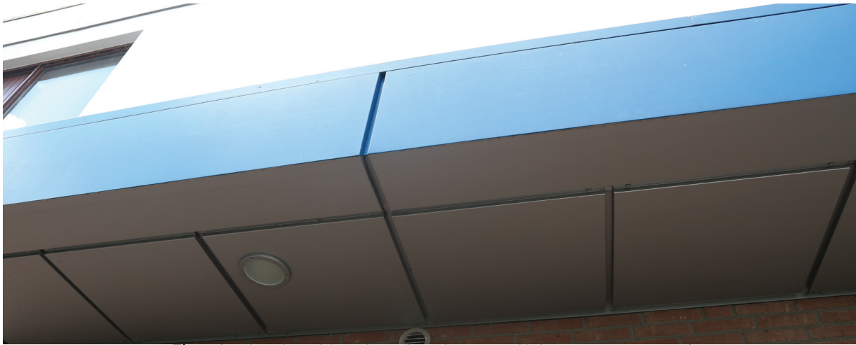
Fig. 48: Alucobond facade Multatuli weg, Delft (source: own image)
