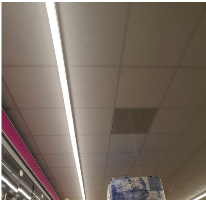
Fig. 57: Drop ceiling, Lidl multatuliweg Delft (source: own image)
