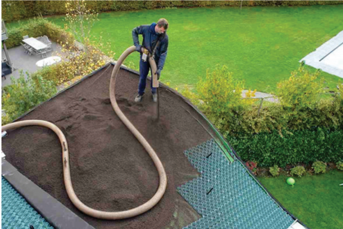
Fig. 88 : Sedum roof laying (grön, n.d.)
