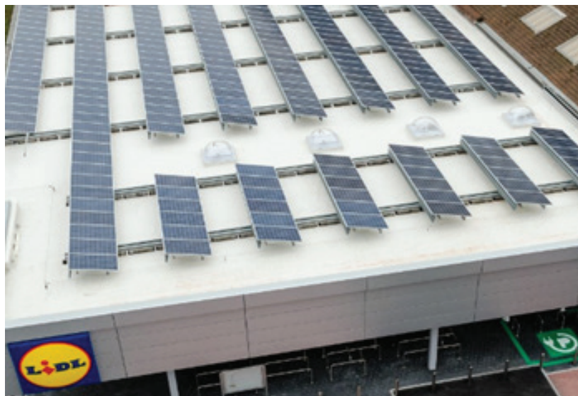
Fig. 79 : Lidl roof, with added solar panels(van Rompaey, 2016)
