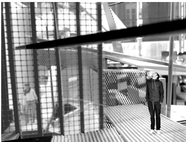
14. Suspended 'columns' attached to a steel hollow steel panel, blurred layers
