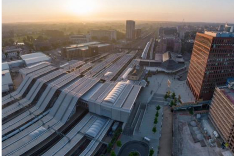
View of Reading Train Station towards London (image courtesy to Reading Gov.)
