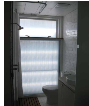
FIGURE 6.65 Translucent thermal storage wall of the Solar Decathlon House 1 of Ohio State University. This thermal storage wall is constructed from two translucent plates of polycarbonate holding water-filled acrylic tubes in-between. This configuration allows sufficient natural light to enter the bathroom and still maintains privacy. Reprinted from Ohio State University website.
