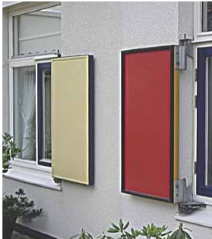
FIGURE 6.2 External hinged thermal shutters. Minimum-energy dwellings, Schiedam, the Netherlands by Jón Kristinsson. Photo by Jón Kristinsson.
