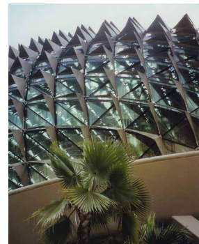
FIGURE 6.47 Fixed iconic shading elements; Esplanade, Singapore by DP Architects.
