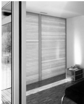
FIGURE 6.66 Translucent window system with thermal buffering capacity from prismatic elements and embedded PCM. Alterswohnen in Domat/EMS, Switzerland by Schwarz Architekten. Adapted from Swiss Solar Agency (2006).
