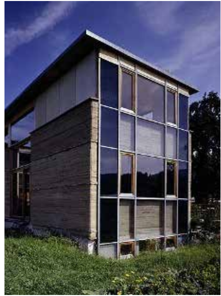
FIGURE 6.23 A spandrel wall executed as a loam thermal storage wall, here flanked by solar cells. The façade also contains windows to admit direct sunlight and provide views outside. Wohnhaus M by Martin Rauch and Robert Felber. Reprinted from Lehm Ton Erde website.
