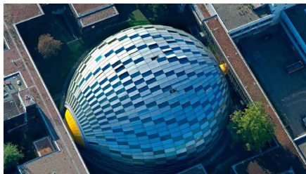
FIGURE 6.55 The double layer of the dome provides solar-induced natural ventilation; Philology Library, Berlin by Norman Foster. Reprinted from Foster + Partners website.
