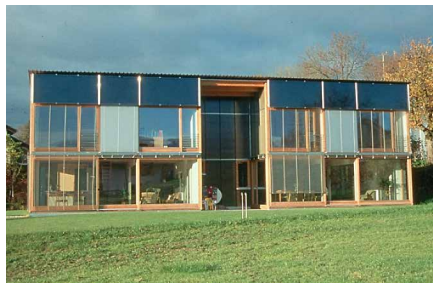
FIGURE 6.16 The sun-facing façade is almost completely transparent. Semi-detached passive houses in Bregenz, Austria by Walter Unterrainer. Reprinted from Walter Unterrainer Architektur Atelier website.
