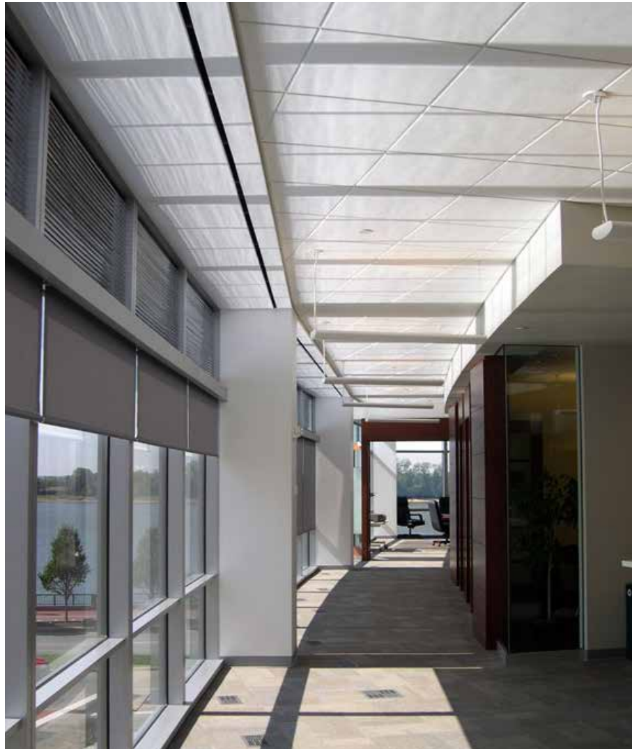
FIGURE 6.39 The LightLouver is a light shelf solution of minimal proportions which makes it easy to use in renovation projects. Old National Bank headquarters, Evansville, United States by HOK. Photo by LightLouver Daylighting System – Copyright 2002, Michael J. Holtz, LightLouver LLC.
