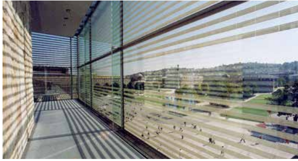
FIGURE 6.48 Printed horizontal lamellas; Stuttgart Museum of Art, Stuttgart, Germany by Hascher Jehle Architektur. Reprinted from Hascher Jehle Architektur website.
