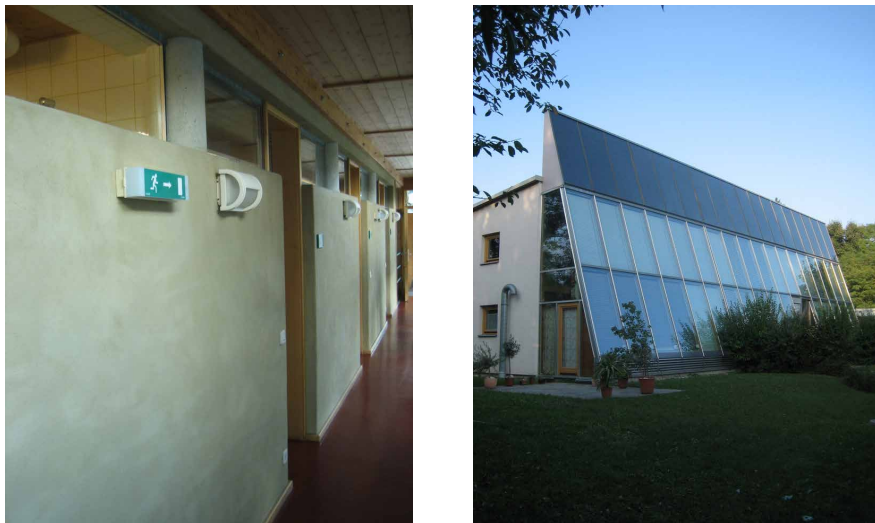
FIGURE 6.11 Thermal mass wall made of loam in AEE INTEC office building, Gleisdorf, Austria.
