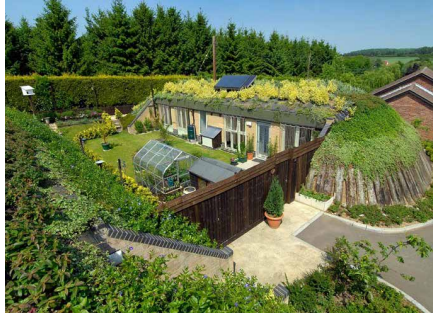
FIGURE 6.32 Honingham Social Housing, United Kingdom by SEArch architects is constructed at surface grade with a bank of earth bermed to its outer walls. Reprinted from SEArch architects website.
