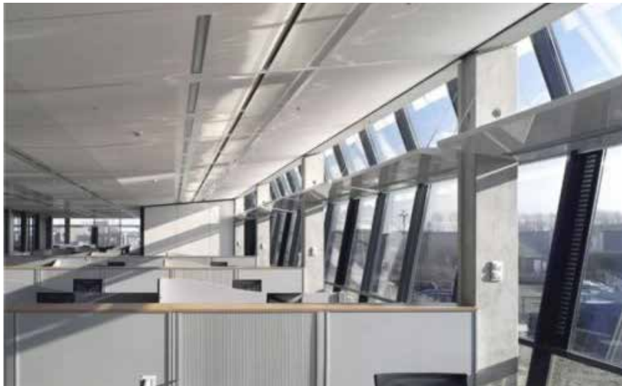
FIGURE 6.43 Light shelves allow natural light to penetrate deeper into the room and reduces bright light levels directly near the window. The light shelves are placed inside the façade to keep the reflective top cover clean (and thus more reflective). The shelves still are pushed to the outside to catch more light, poking the building envelope outwards. Amgen office building, Breda by Ector Hoogstad architects. Photo by Marcel van Kerckhoven.
