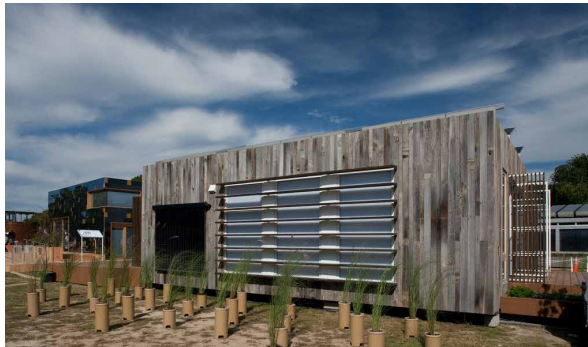
FIGURE 6.65 Translucent thermal storage wall of the Solar Decathlon House 1 of Ohio State University. This thermal storage wall is constructed from two translucent plates of polycarbonate holding water-filled acrylic tubes in-between. This configuration allows sufficient natural light to enter the bathroom and still maintains privacy. Reprinted from Ohio State University website.
