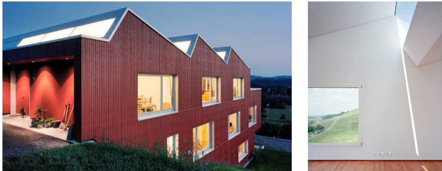
FIGURE 6.37 House Uesslingen by Spillmann Echsle Architekten features a saw tooth roof with skylights to allow more daylight into the building. Photo by Spillmann Echsle Architekten.
