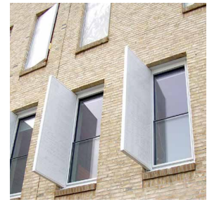
FIGURE 6.64 Externally hinged thermal shutters that function as a shading device. Municipality office in Bronckhorst, the Netherlands by Atelier Pro. Reprinted from Atelier Pro website.
