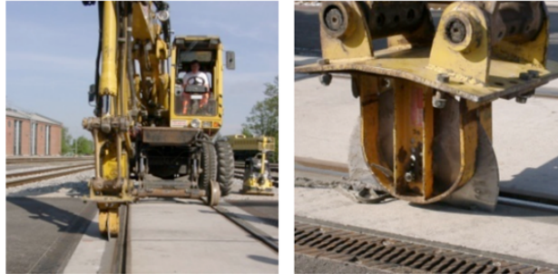
Figure 21 Removal of Corkelast® resin in the rail replacement (edilon)(sedra, 2018b)
