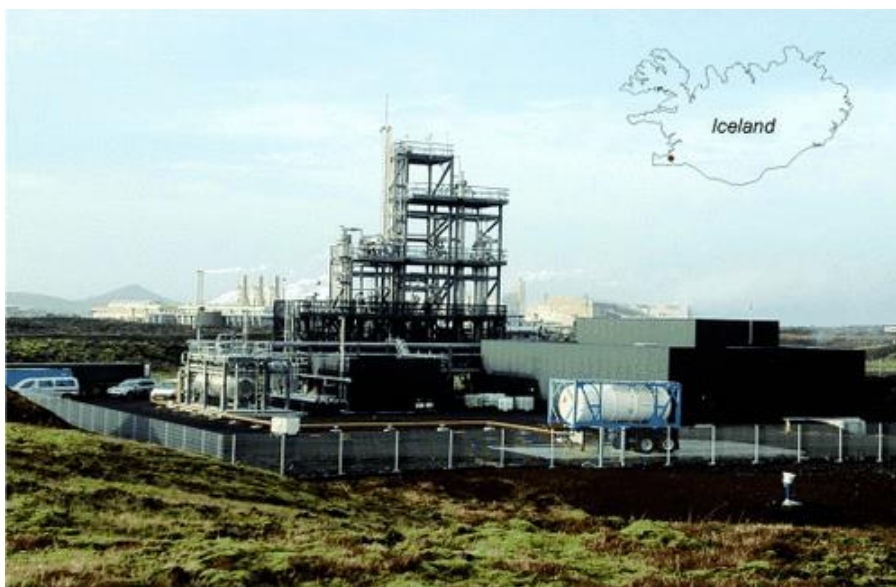
Figure 1.2 The “George Olah Carbon Dioxide to Renewable Methanol Plant” of Carbon Recycling International in Iceland based on local geothermal energy. The first commercial carbon dioxide recycling plant operating in the world. 7
