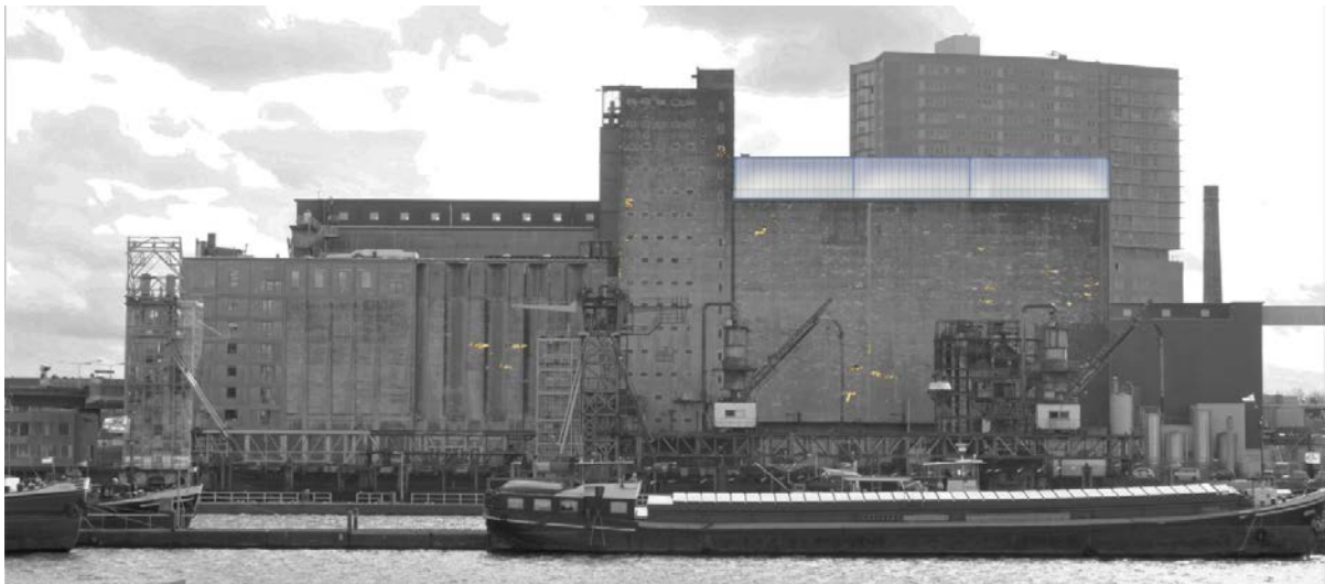
North façade intervention roof and façade. Own image/photo
