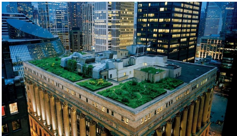
Figure 2.7 The rooftop garden at Chicago's City Hall. DJANDYW.COM
