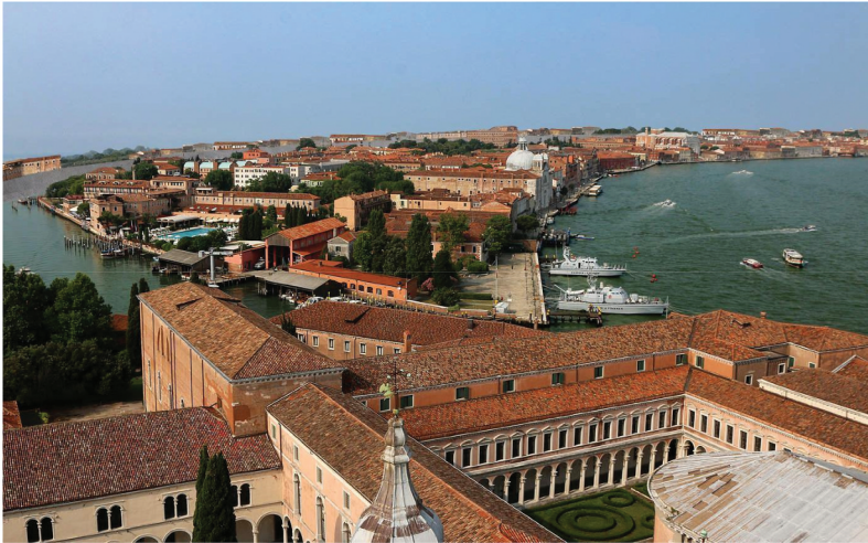
Figure 7. The symbiotic system design proposal. View impression of new developments and integration of the dam-ring into the current urban tissue of Venice (Buis et al. 2021).
