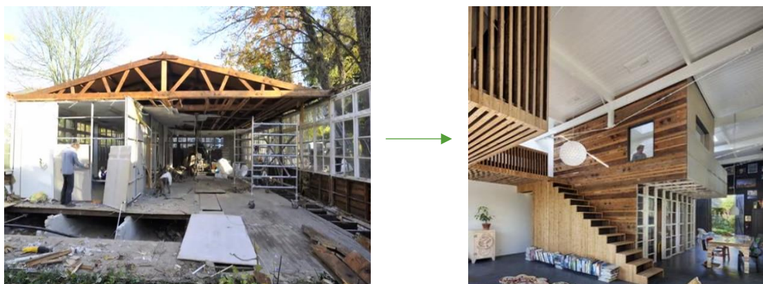
Figure 8: House of Rolf, materials from the building in the right picture were used for the construction of the interior of the house (Bruggink, 2014).
