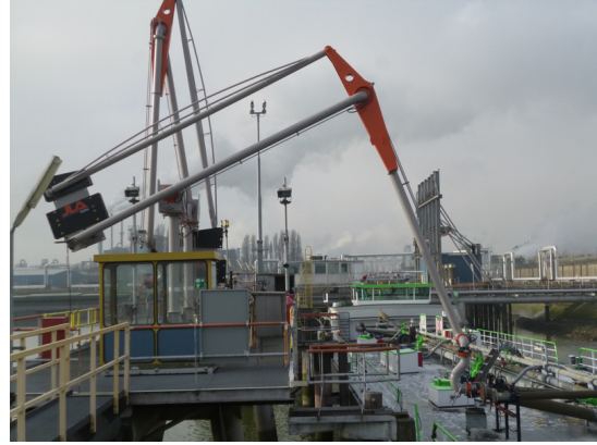
(b) An example of a loading and unloading arm for ammonia with a ship [39]
