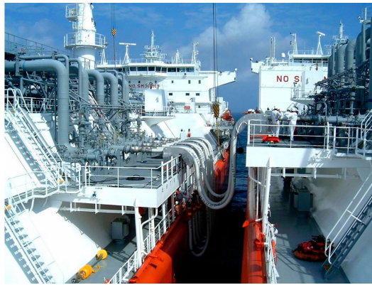
(c) An example of a loading and unloading connection for ammonia with ship to ship loading [9]
