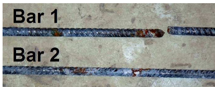
Figure 4-28: Reinforcing bars of the RC beams of Test 1A. Bar 1 was the reinforcing bar of the chloride-exposed beam. Bar 2 was the reinforcing bar of the beam exposed to tap water.
