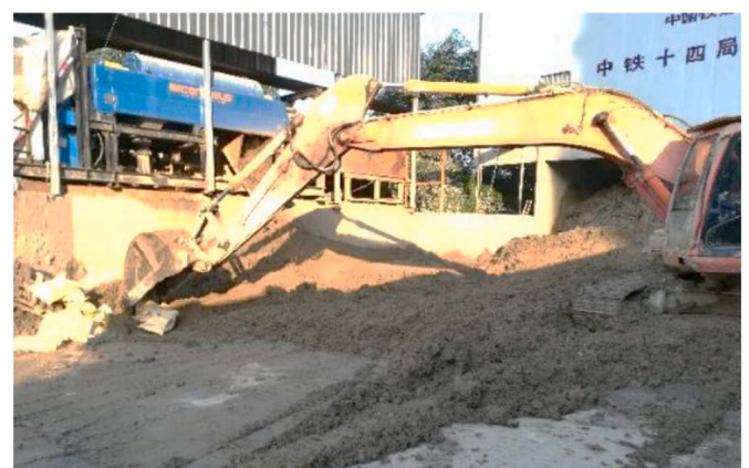
Fig. 15. Stockpiling of discharged soil from shield tunnel construction (Zhang et al., 2022a).
