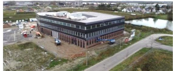
Figure 13: overview of building after construction (photo DVV)
