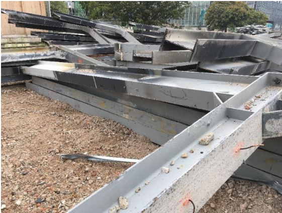
Figure 9: improper storage of donor steel after demolition
