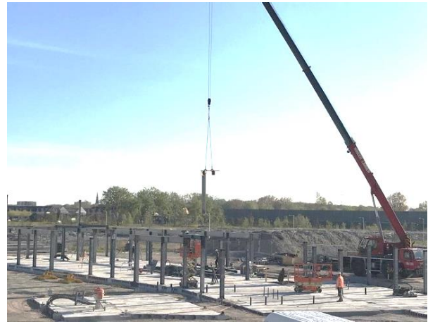
Figure 11: Assembly of steel elements (photo: De Vries en Verburg contractor, DVV)
