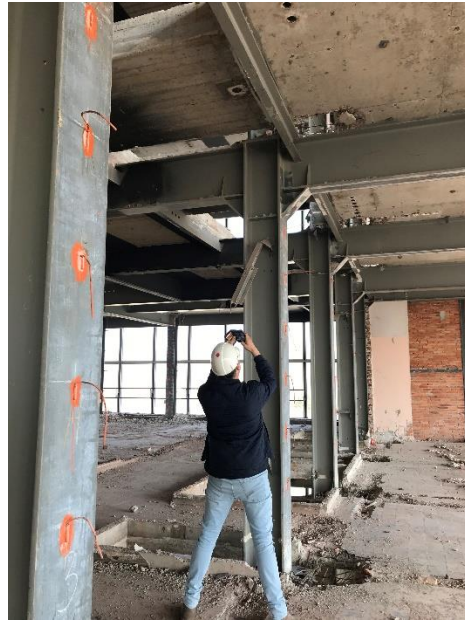
Figure 7: steel elements in the existing building, during inspection
