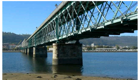
Fig. 3. Eiffel bridge – Viana do Castelo, Portugal [43].
