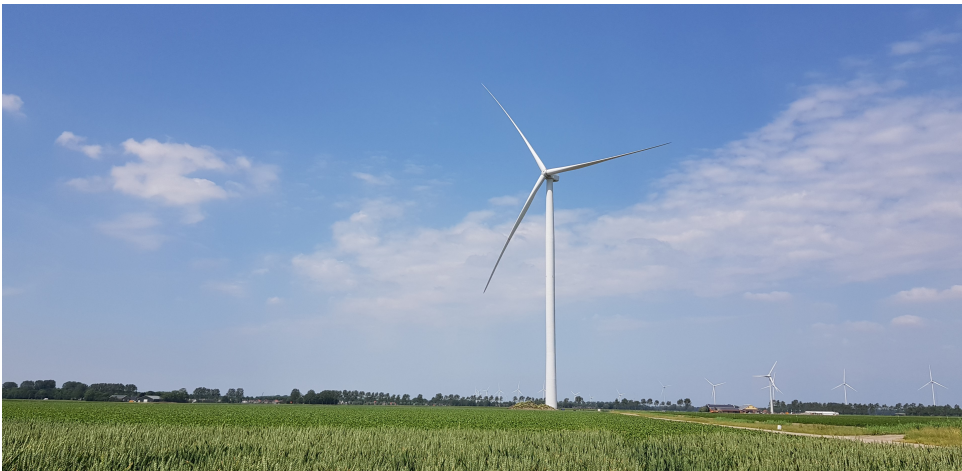
Figure 5.13: The TIADE research turbine in Wieringermeer, North Holland, Netherlands
