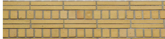
Figure 7: Masonry bond (Flickr, 2010)
