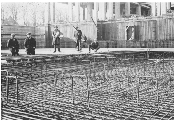
Figure 6: Construction of reinforced concrete (n.a., 1931)
