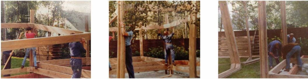
FIG. 5.9 Pictures of the prototype's building process. Source: VAI
