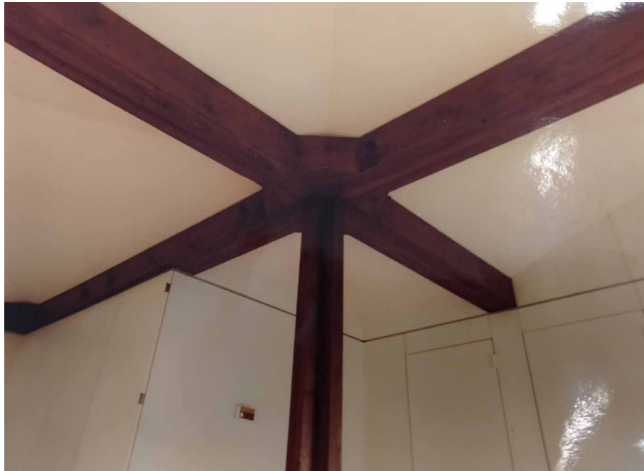
FIG. 5.16 The knooppunt as seen in the interior of the 78+ prototype. Source: VAI.
