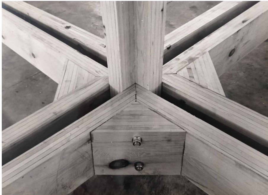
FIG. 5.7 Photograph of the knooppunt assembly. Source: VAI
