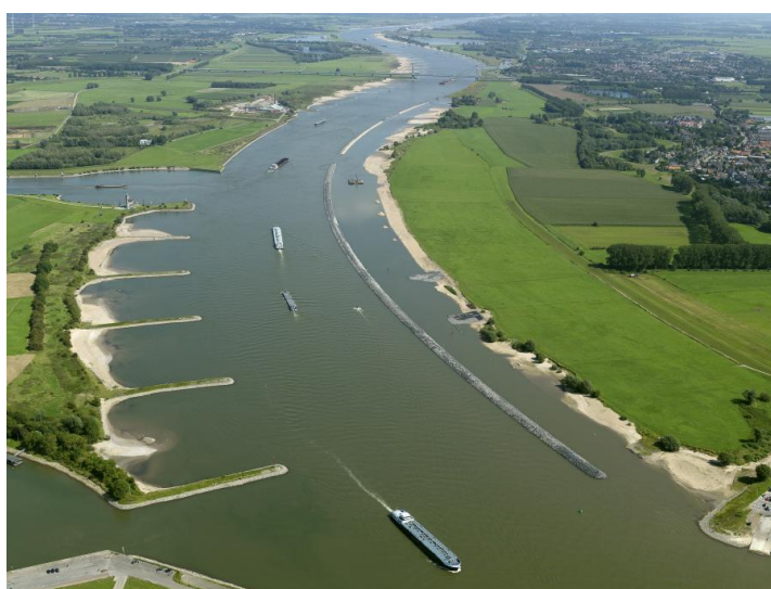
Figure 1.1: The longitudinal training walls in the Waal near Wamel. The longitudinal training walls are located in the inner bend and groynes in the outer bend. [Your Captain Luchtfotografie]
