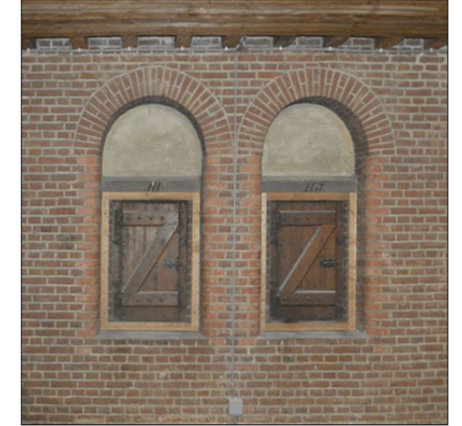
Especially around the window there is beautiful brickwork
