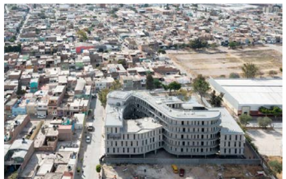
Image 4: Affordable housing development in Mexico
