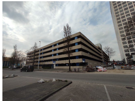
Figure 24 Europoint Parking Garage- Future CMH Location
