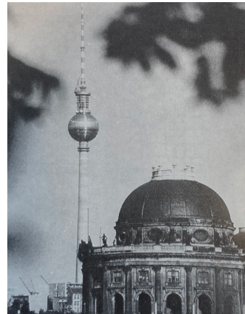
Figure 22. Berlin Television Tower. Source: Berlin und Seine Bauten. (1987)
