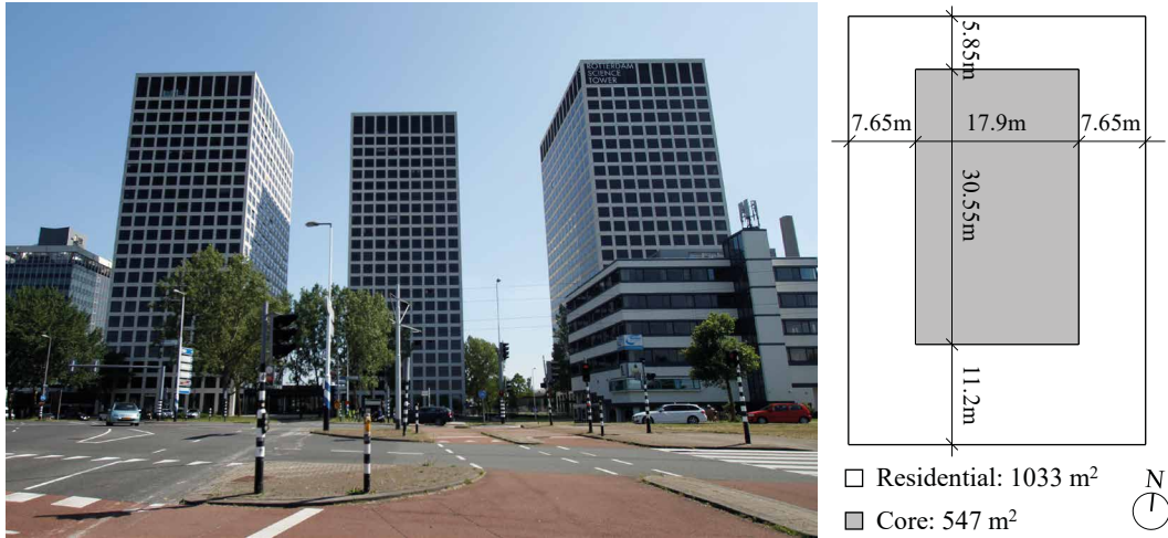
FIG. 5.2 Europoint complex in Rotterdam, the Netherlands
