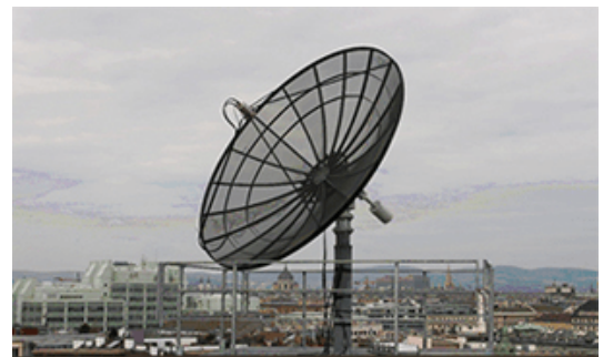
Figure 10.1: Parabolic antenna at Vienna University of Technology for downlink in S-band [60].
