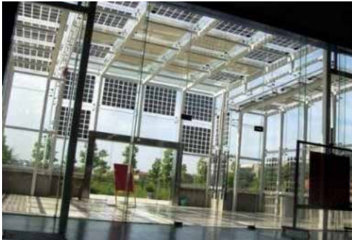
(a,b) Examples of two applications with c-Si solar modules (Building Constructions 2020)
