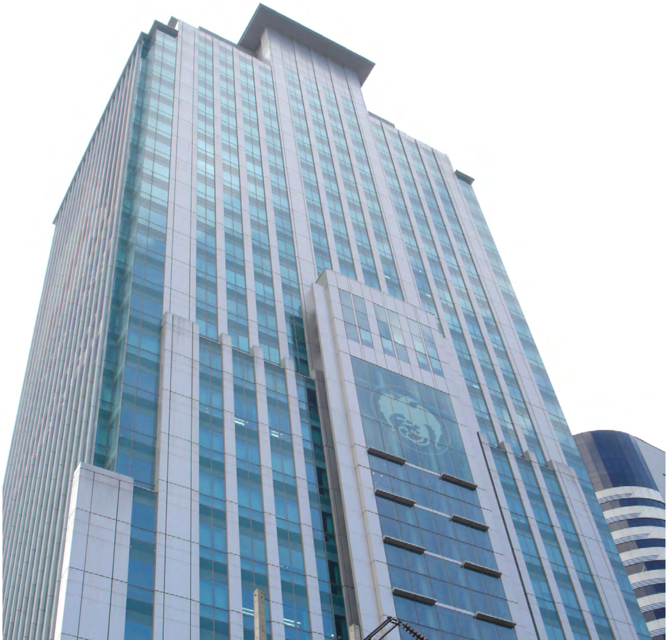
Figure 6-2 : Krungthai Bank - Sukhumvit Building's East facade
