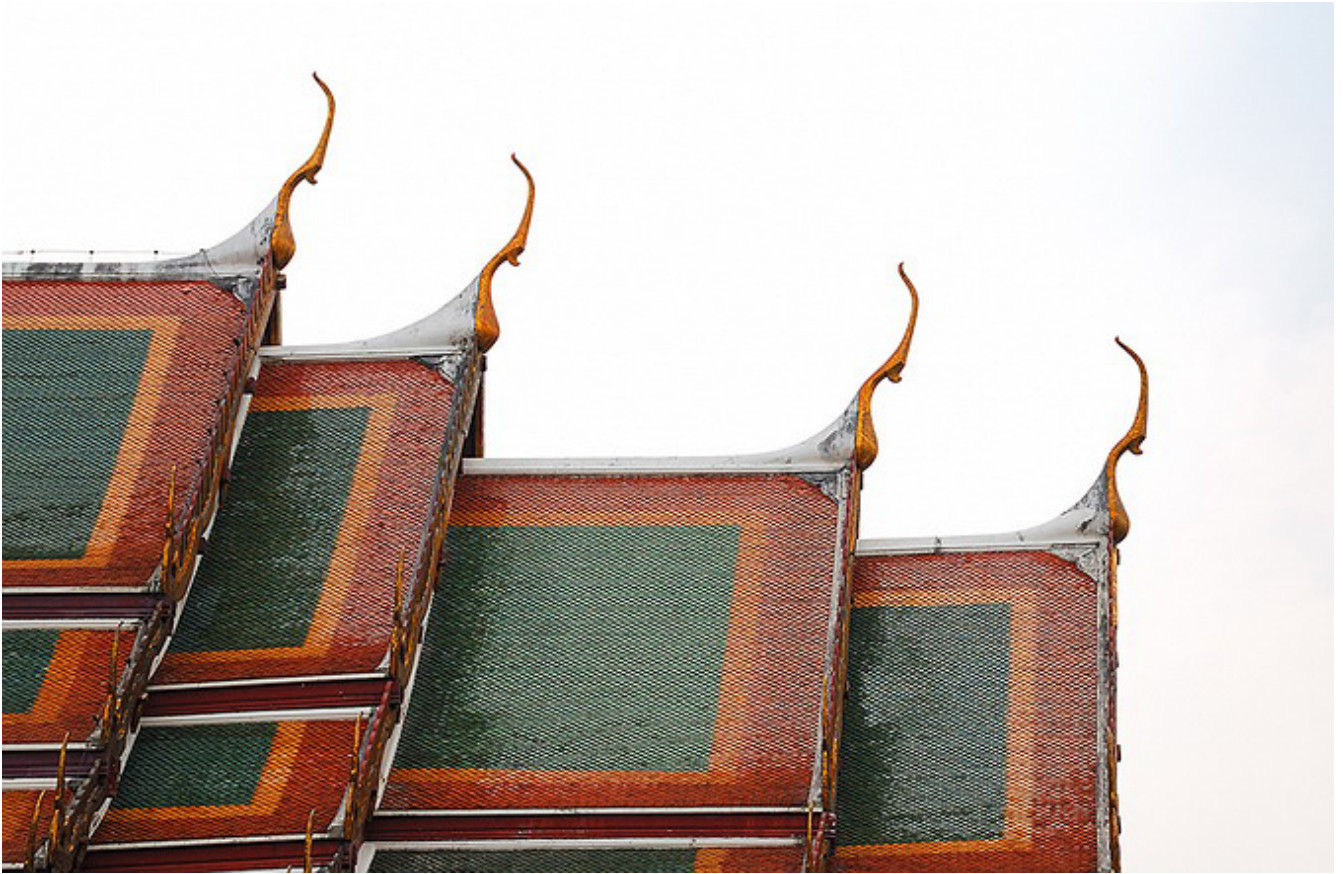
Figure 8-1 : Multi-tier roof design technique used to create the buoyancy effect in Thai temple.
