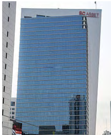
Fig. 2-37 Shinawatra III Tower
