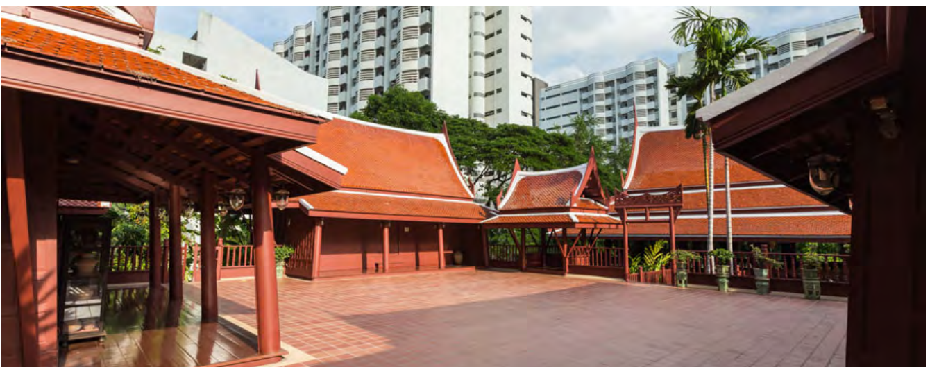
Figure 5-4 : 'Chaarn' or large balcony connecting a group of houses. Chulalongkorn University. "Chulalongkorn Thai Building" Chulalongkorn University, http://www.prm.chula.ac.th/cen046.html
