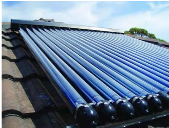
Figure 4-18 : Evacuated tube solar collectors (ETC) (Tyagi et al., 2012)
