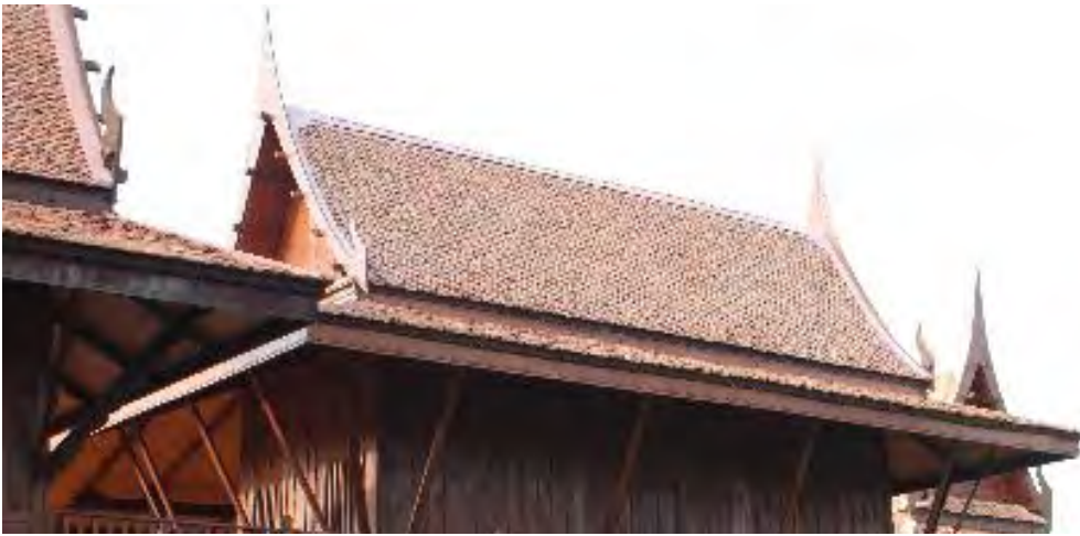
Figure 5-6 : Extended Roof of a traditional Thai house.
