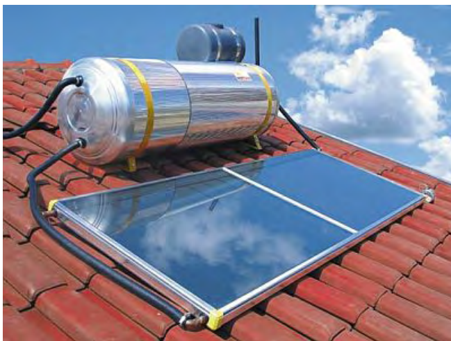
Figure 4-17 : Flat plate solar collector (Tyagi et al., 2012)
