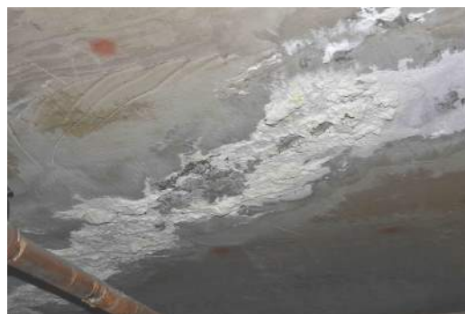
Figure 6.1: Efflorescence (Hering, 2012)
