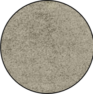
EXISTING CONCRETE CLADDING
