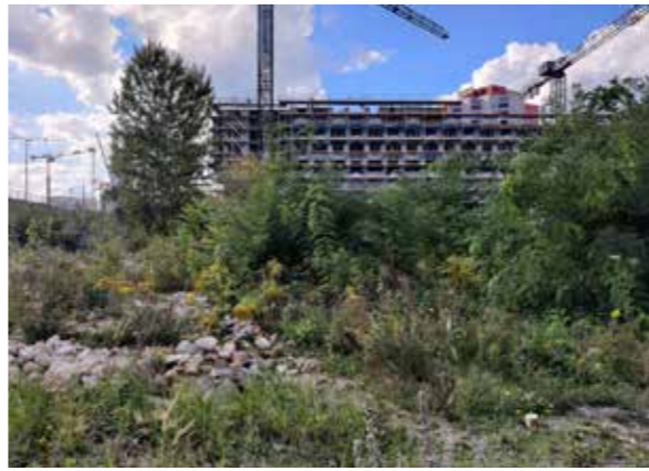
CONSTRUCTION TO THE WEST
