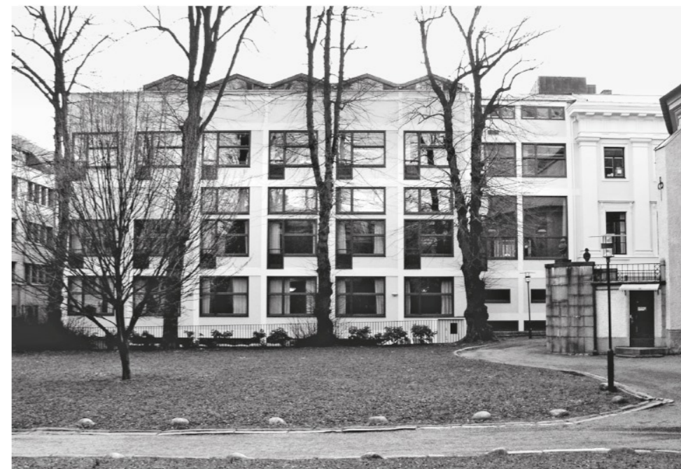
Photograph of the west facade. Adams, N. (2015).
