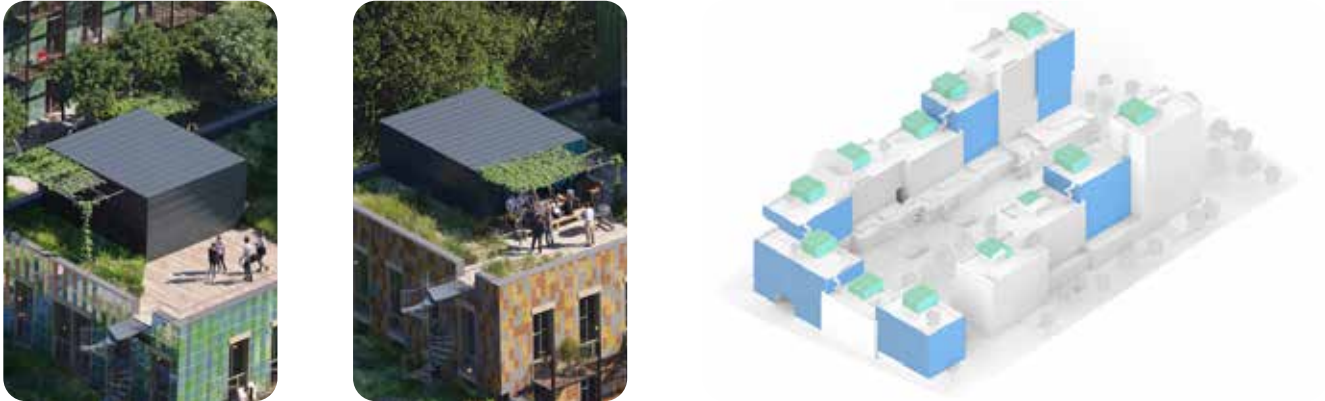
Figure: Mad Arkitekter (2019). Solar-powered facades and PV panels on the roof.
