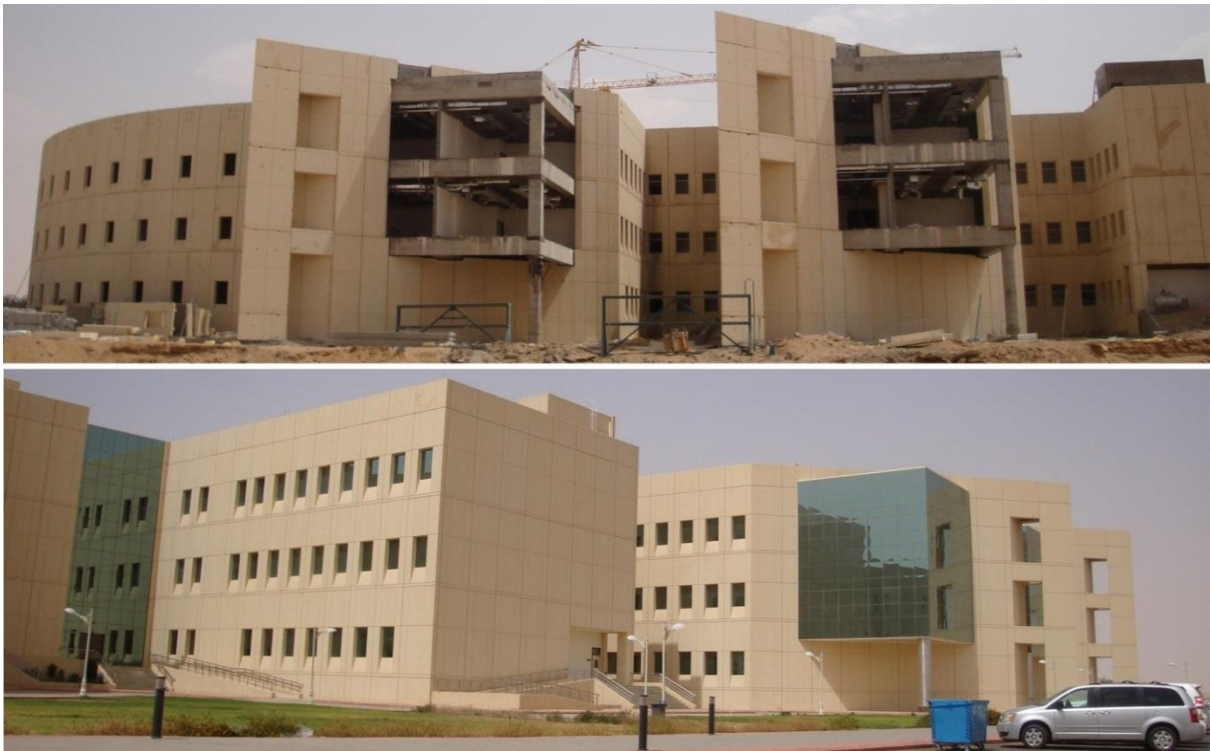
Figure 4.24: The use of pre-cast concrete in Najran University
