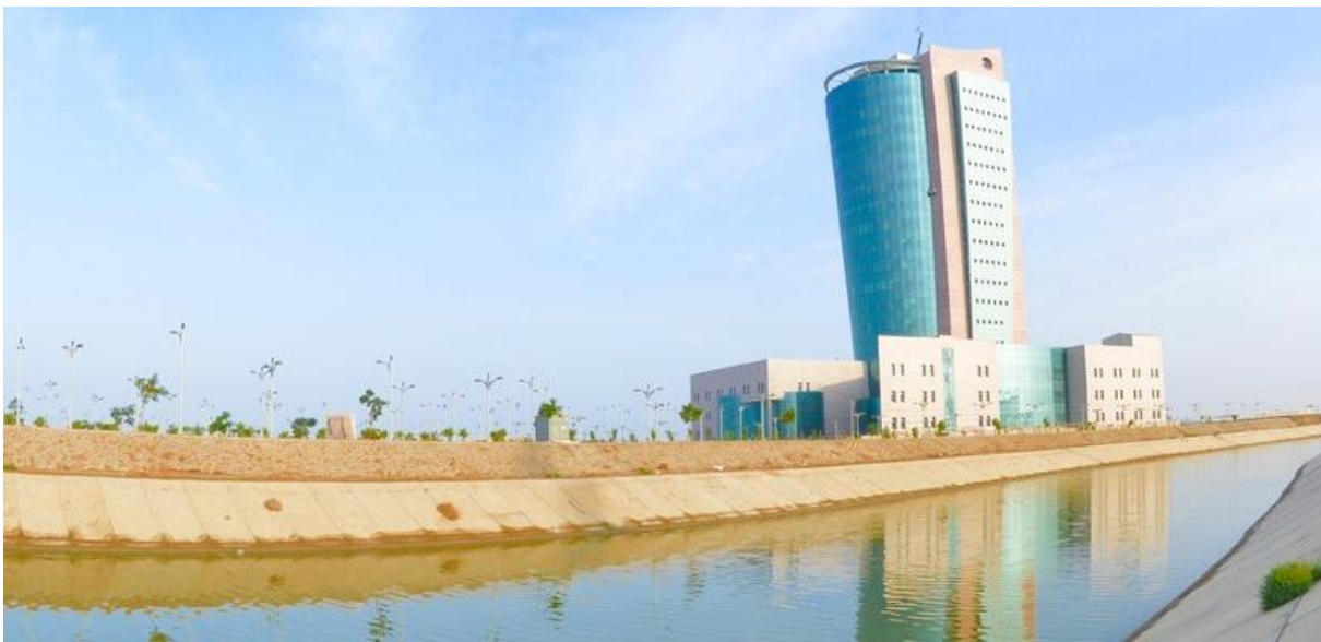
Figure 4.7: Jazan University Admin. Tower (Jazan University 2017)
