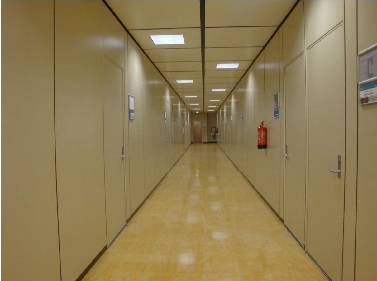
Figure 4.61: The metal floor-to-ceiling partition system in King Saud University (KSU)
