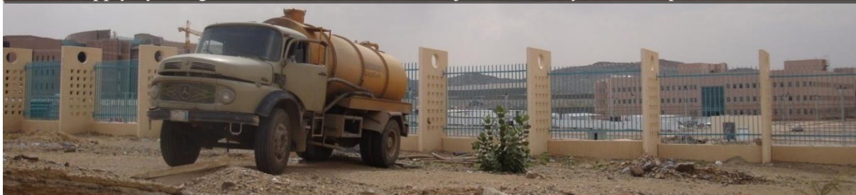
Septic tanks are emptied by vacuum truck in Al Baha University, southern part of the KSA
