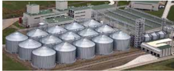
Big scale stainless steel silos (SCAFCO Commercial Grain Bins & Silos 2015)
