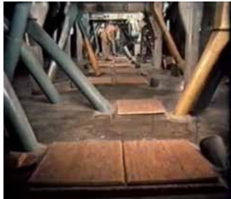
5. The distribution floor with the pipes that let the grain into the silos
