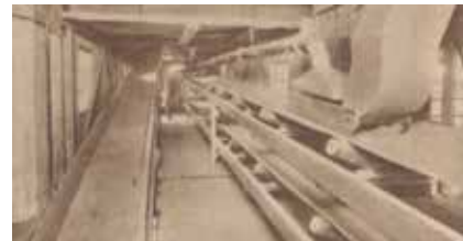
Distribution floor (Maaslandse Courant 1930)
