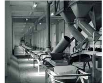
Horizontal conveyor in the postma part (CV Maassilo. 1951)
