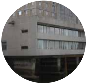
Due to lack of space on the land they placed the office on the waterside in 1964
