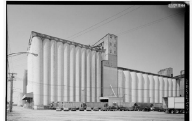
American Elevator made out of concrete Buffalo, New York built in 1906 ( http://wikimapia.org/12904236/American-Elevator )
