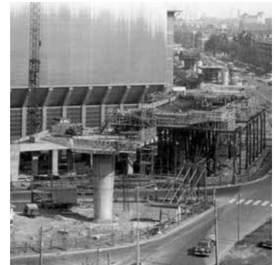
The metro station under construction (Cees Schultz, 1965)
