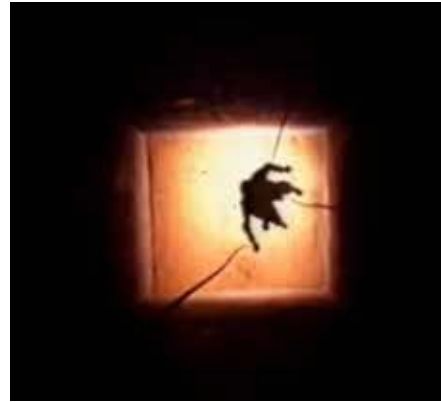
6. Inspector goes (rarely) into the silo
