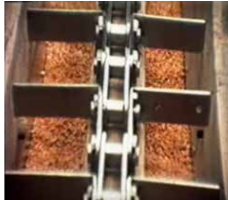
2. The elevator leg transport the grain to the distributing floor
