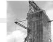
New facade elevator tower
