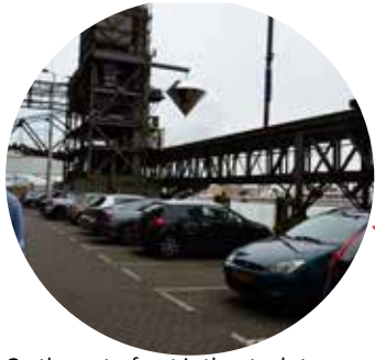
On the waterfront is the steel structure placed, that bridge the connection from the boat to the Maassilo. This structure is part of the machine and is not in use anymore
