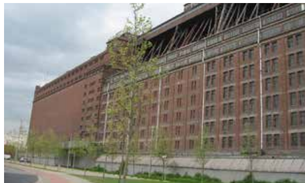
Silo made out of bricks at the harbor of Bremen build between 1914 and 1929 ( http://corabuhlert.com/2013/05/18/photos-bremen-harbour/ )
