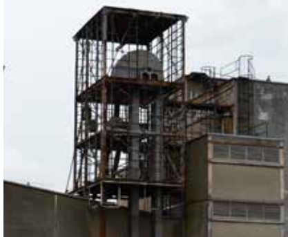
Vertical elevator on the roof (Bronswijk, B. 2016)
