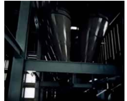
8. At the top of the work floor you see the funnels of the silo
