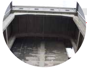
The bridge construction build on top of the transformation plant
