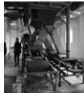
Relics of former machinery
