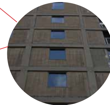
The expression of the structure with the infill of tiles motif
