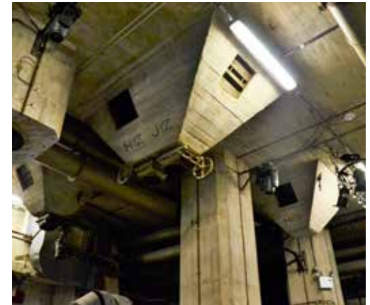
Ceiling of the work floor of the Maassilo
