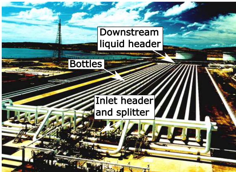
Figure 1.2: Example of a slug catcher with 5000 \text{ m}^3 liquid storage volume. Adapted from [39].
