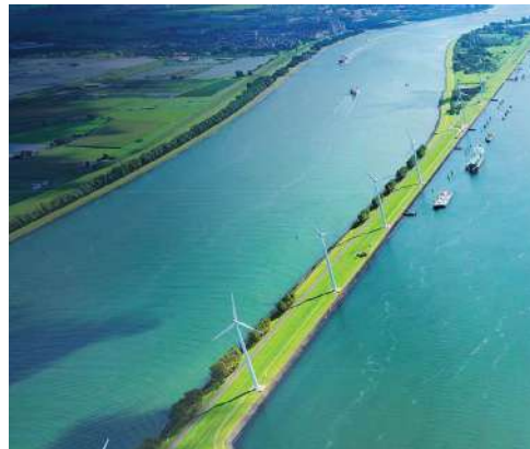
Wind energy system
