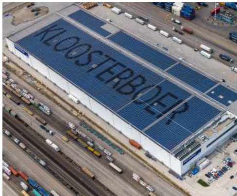
Solar energy system
