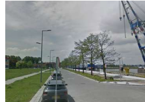
D. Eemhaven Linear green spaces alongside the road are adjacent to the river
