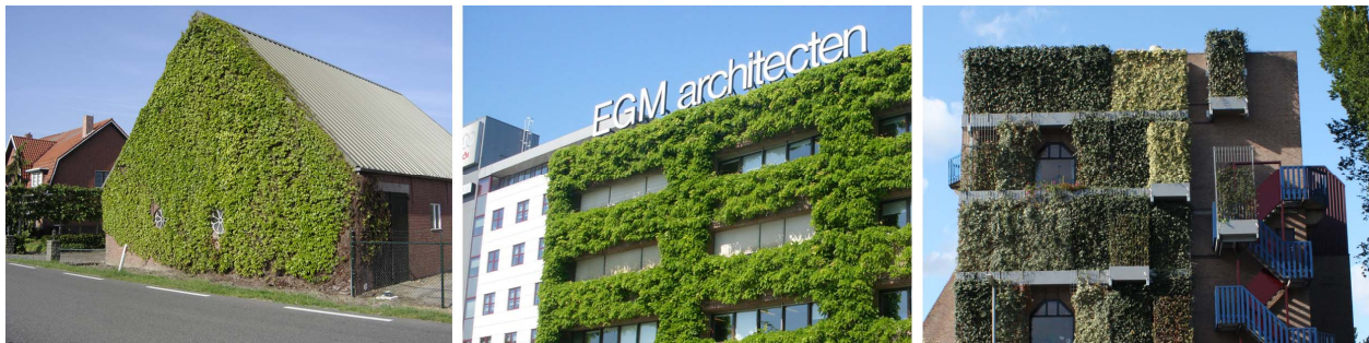
Figure 4. Direct greening system (a), indirect greening system (b), indirect greening system combined with planter boxes (c).
