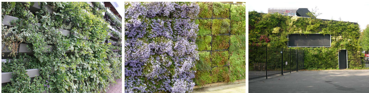
Figure 5. LWS based on planter boxes (d), LWS based on foam substrate (e), LWS based on felt layers (f).
