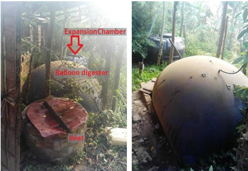
Figure 20. Balloon type digester
